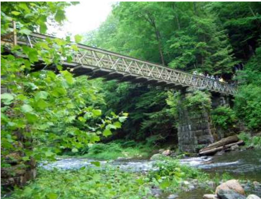
The Mahican Mohawk Trail crosses South River on old railroad abutments. Credit: L.Stevens
