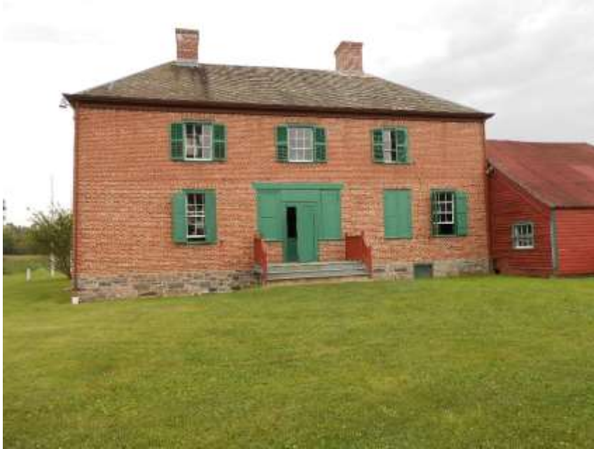
The c. 1788 Knickerbocker Mansion as rehabilitated in Schaghticoke. Credit: L.Stevens
